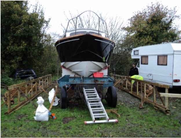
Setting up the sills
