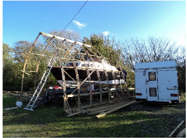
Erecting the frames
