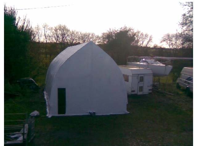
The finished shed shrinkwrapped
