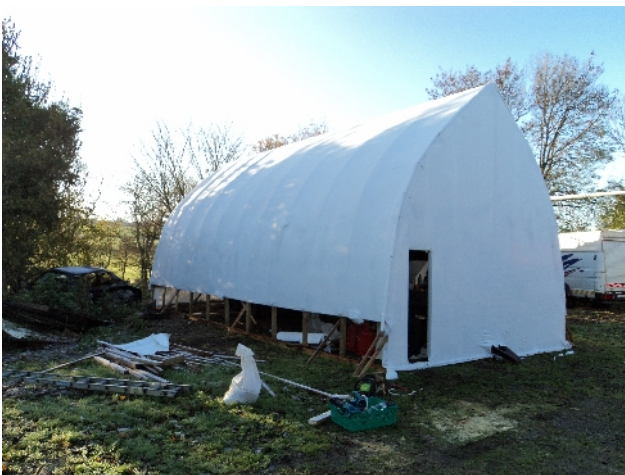
Film attached as far as the sill
