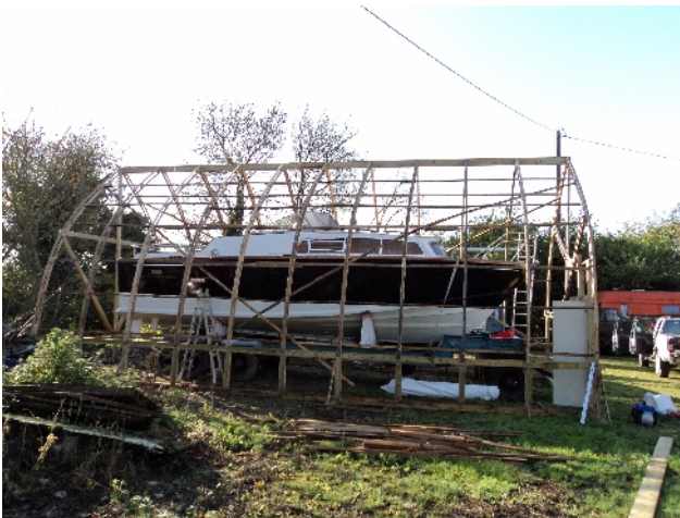
The frames and door fitted
